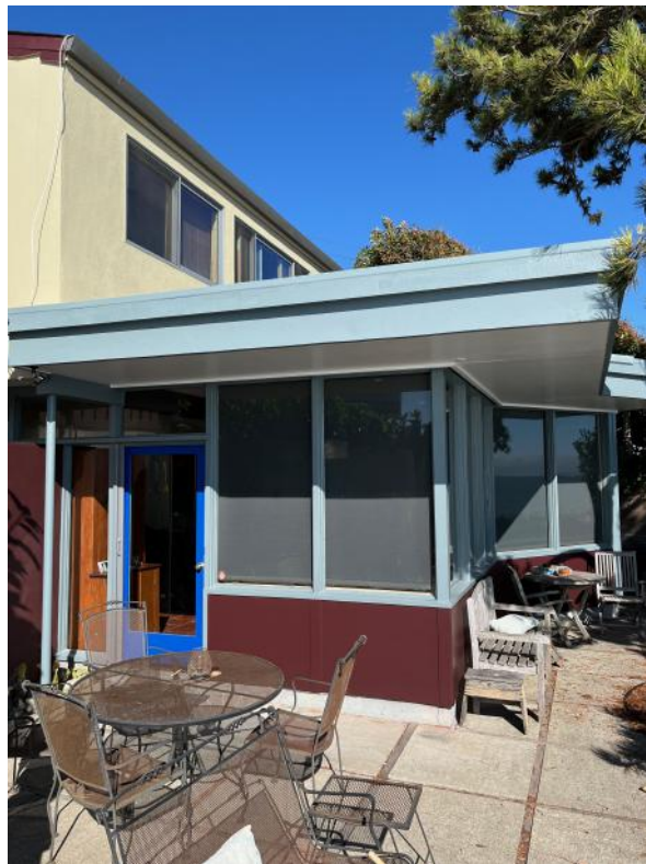
West facade of 1949 living room addition, looking east.
