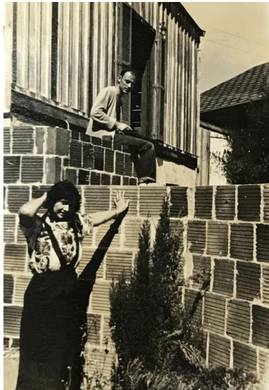
View of rear facade of 771 Ocean Ave., early 1930s. Hollow clay tile wall separating 771 and 775 Ocean Ave. is still unstuccoed. John Haley seated on top of wall. (Haley collection, Richmond Museum of History)
