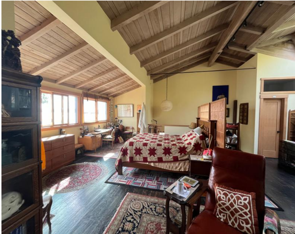
Interior of second floor studio space, looking west. Sleeping porch addition at left.
