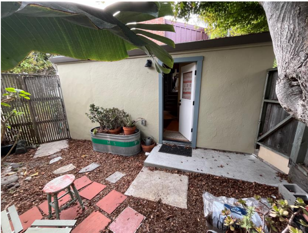
East facade of garage/guest room, looking west.
