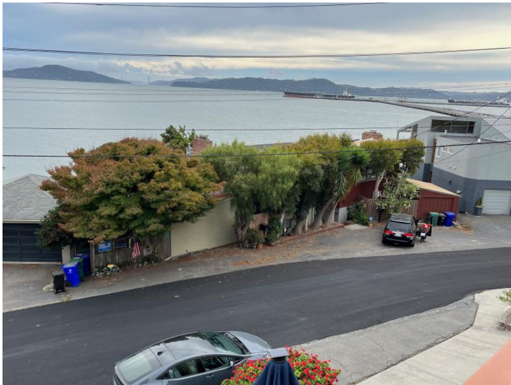
Front (north) facades of 771 (left) and 775 (right) Ocean Ave. looking southwest.
