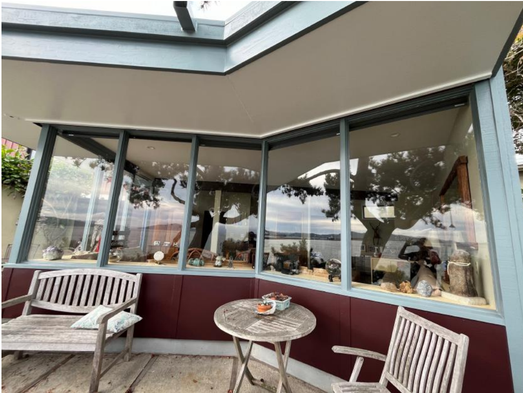
South facade of 1949 living room addition.
