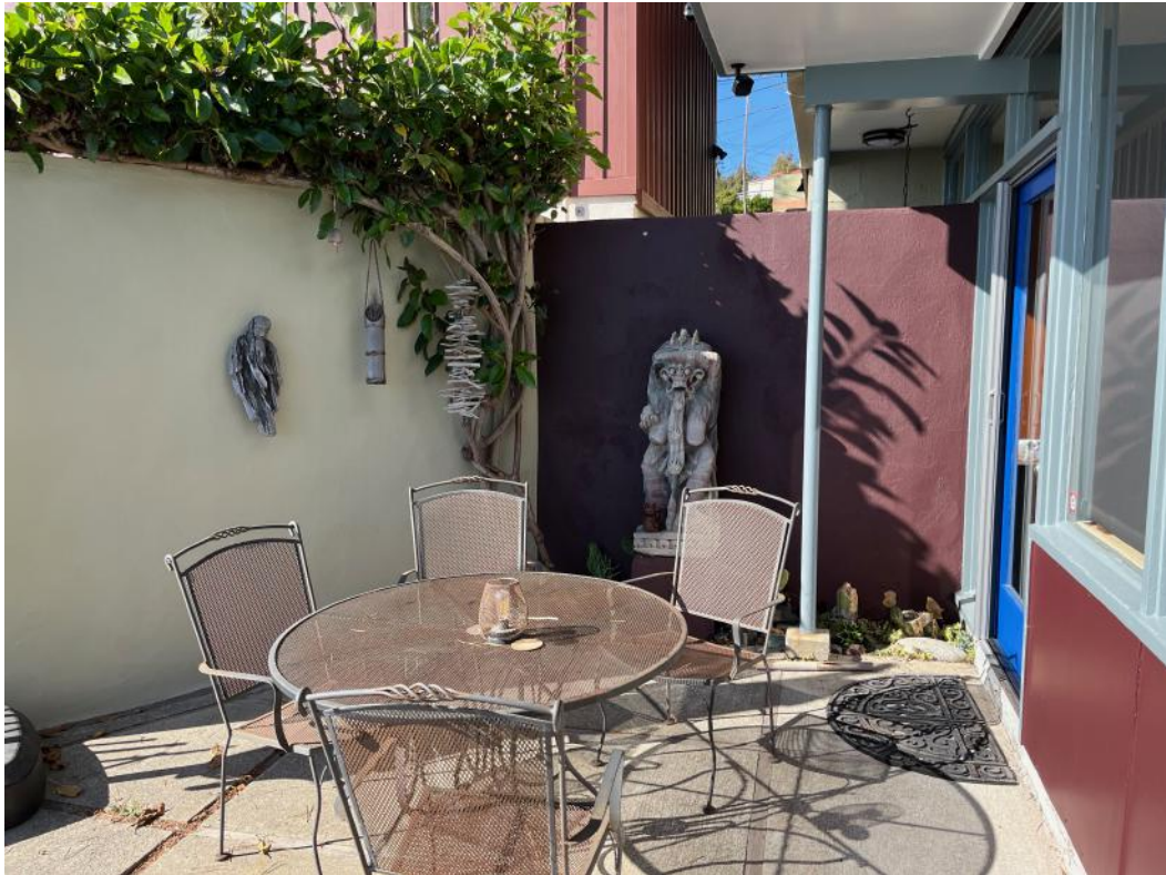
Patio at west side of living room addition. Primary entrance is beyond wall at center. Wall at left/center is hollow clay tile wall that extends into entry and extends south to separate 771 from 775 Ocean Ave.
