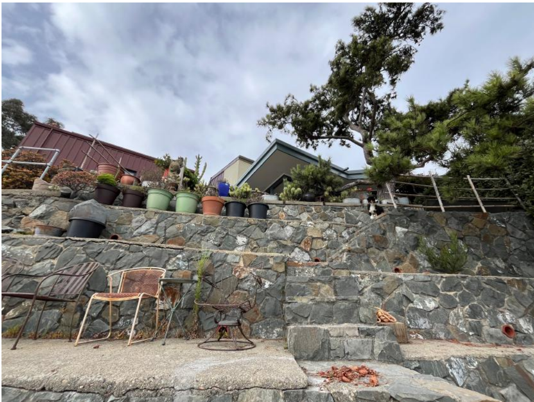
View from lower rear terrace looking up (north) at rear of 775 (left) and 771 (right) Ocean Ave.
