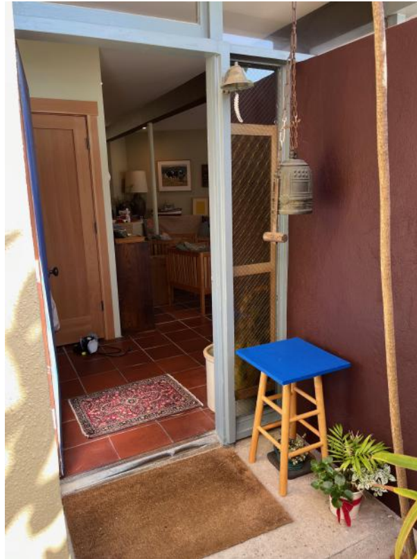
Detail of primary entrance on west facade.
