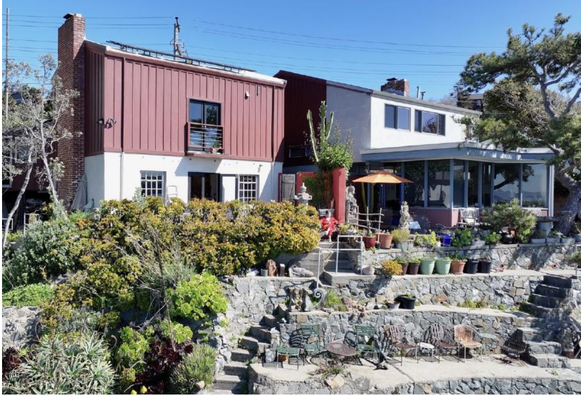
Rear (south) facades of 775 (left) and 771 (right) Ocean Ave. looking northeast.
